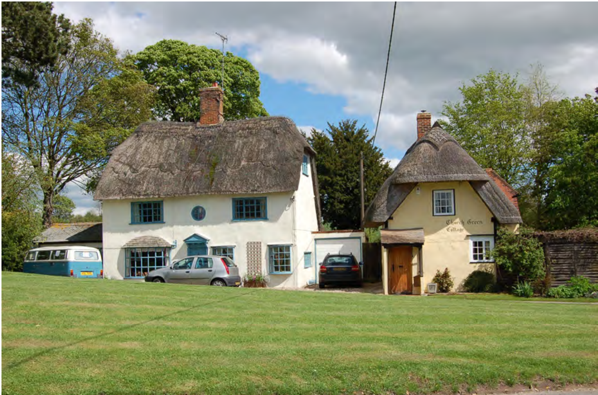
Picture 1.16 A very English scene - Dove Cottage (left) and Church Green Cottage (right) front onto Church Green and are set in scale by mature trees in the background. The presence of utility poles detracts from the quality of this view
